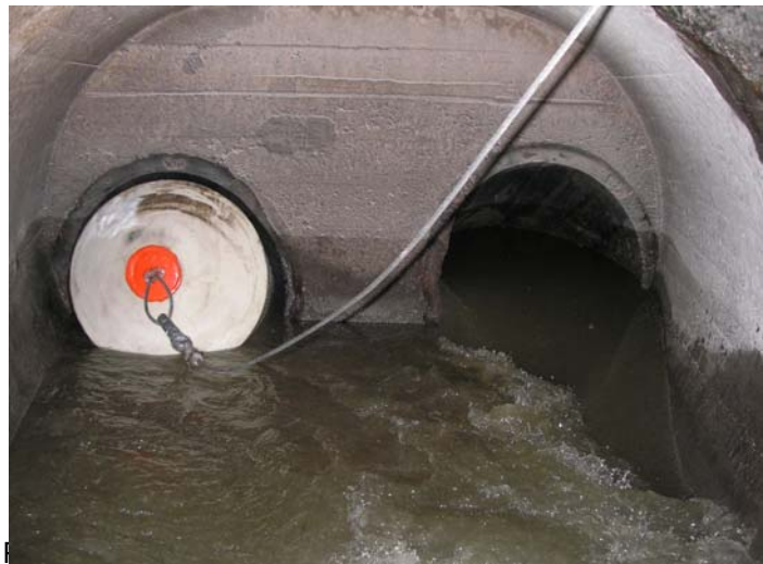
Figure 4 29.5-inch Pig exiting West Siphon
