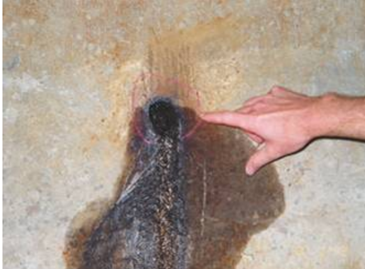
Figure 3. Soil stability checked by cutting small holes in steel plate prior to cutting full sized portal for MTBM launch or retrieval
