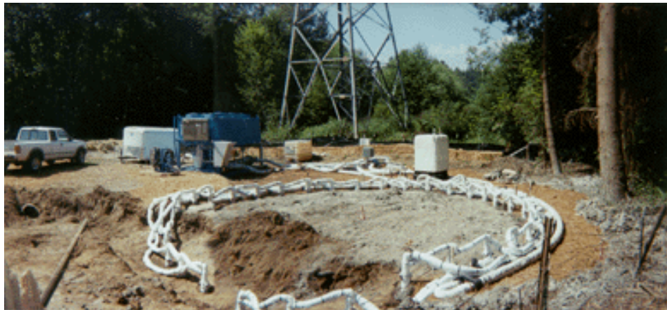
Figure 6. Cooling pipes freezing groundwater prior to shaft excavation ( www.cryocell.com )
