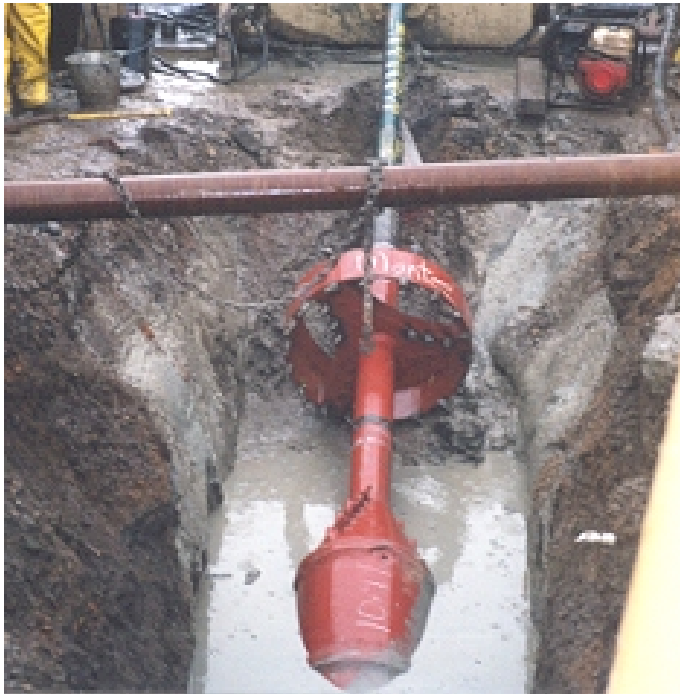
Figure 4 Second Reaming Pass
